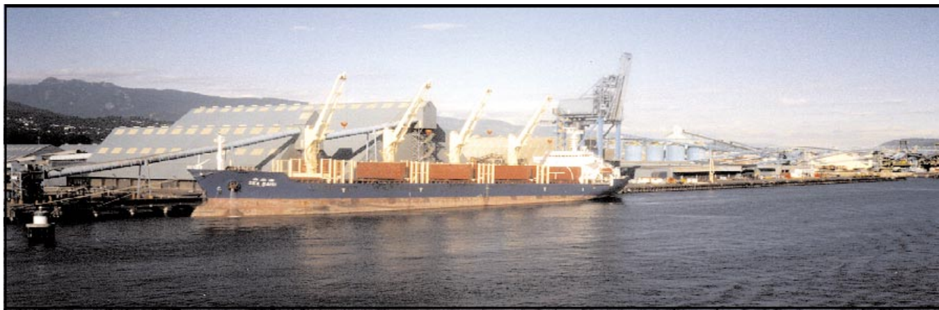
Vancouver Wharves—West Dock
